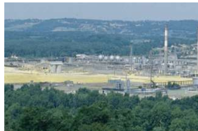
Lacq Gas Processing Facility
