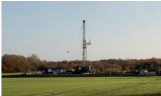
Drilling operations in the UK, 2010.
