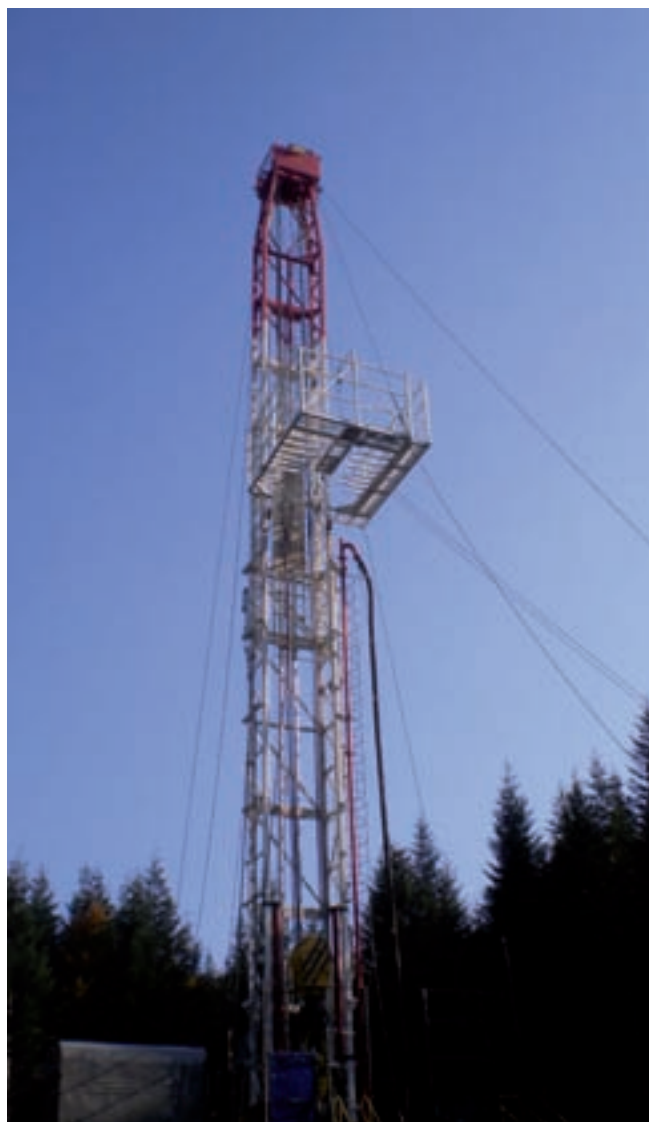
Drilling operations in Romania, October 2010.
